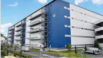
Logistics warehouses operated nationwide
