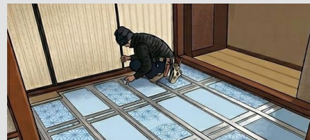
Floor insulation in Single-Family Homes (XPS boards)
