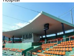
Waterproofing division : Kurume City Baseball Stadium
