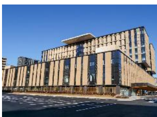
Buildings division : Sendai Kosei Hospital
