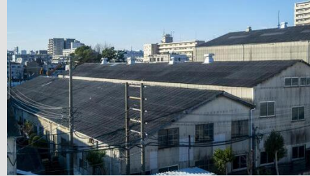
Factories of major building materials manufacturers
