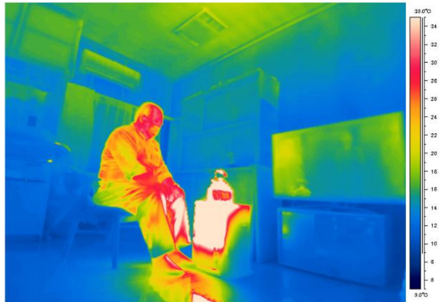
Before insulation and airtightness retrofit
